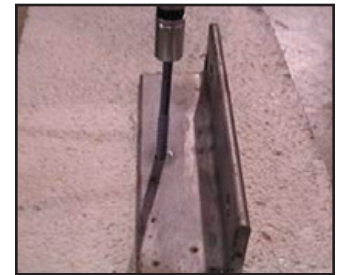
3. Place head of anchor in hex socket, positioning the anchor in the drilled hole, and drive anchor until anchor is fully seated.
