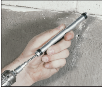
2. Install drive sleeve over drill bit
